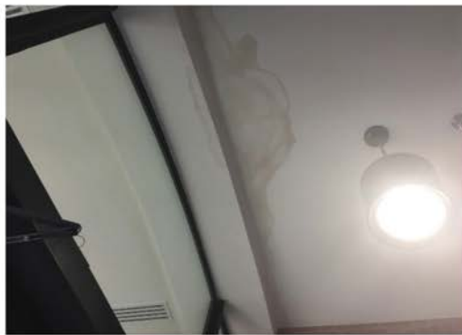
Main entry ceiling leak
