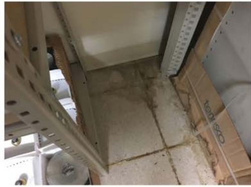
Elect. Room floor leak
