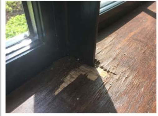
Water damaged window sill
