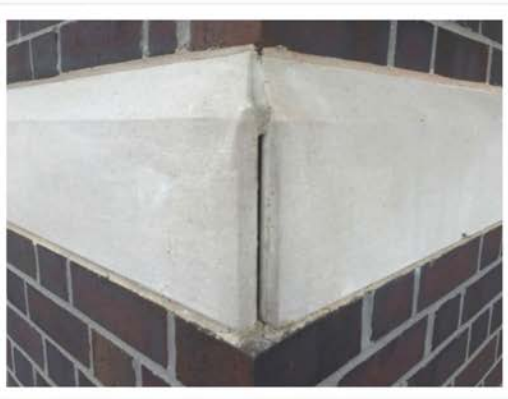
Missing mortar joints
